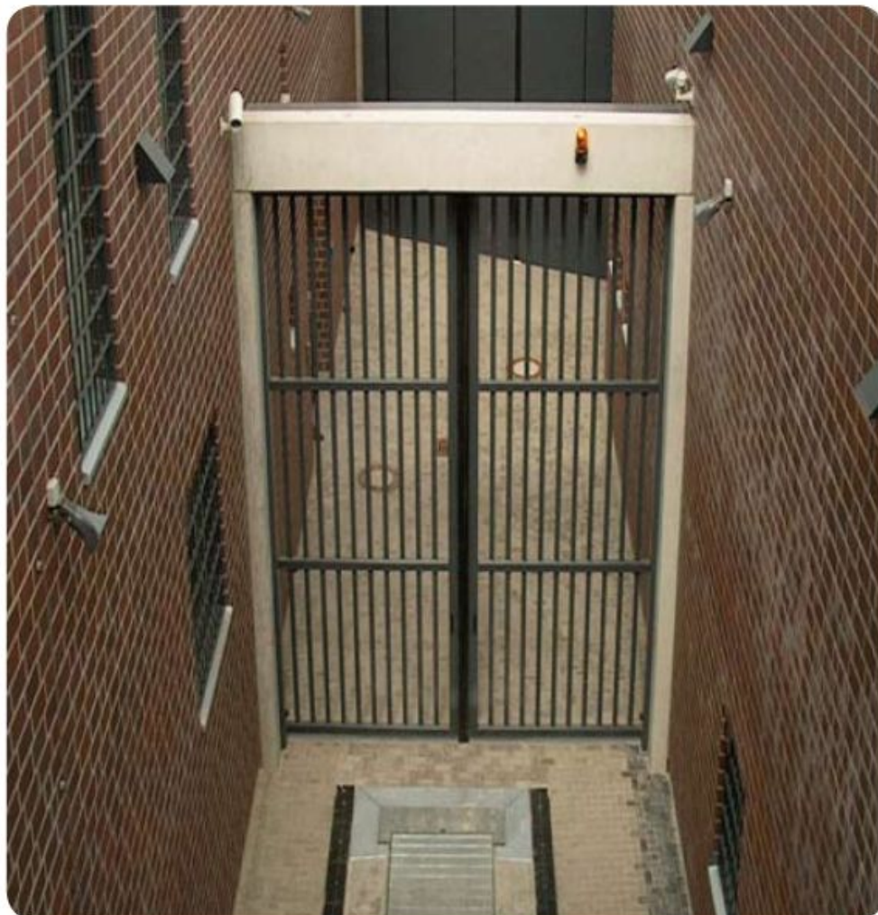
Heavy sliding door situation with truck-ramming-protection
